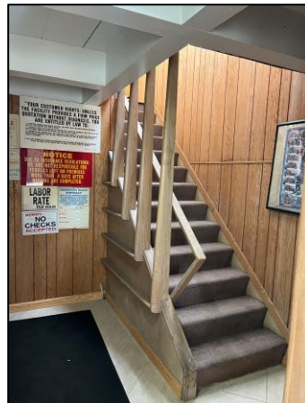
Front Stairs to 2 nd Floor
